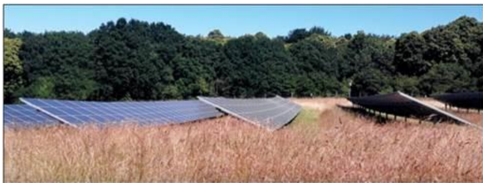
Figure 6: Sites where a “Shade Cut” has been employed during the growing season to prevent shading of panels, but allow flowering meadow elsewhere
